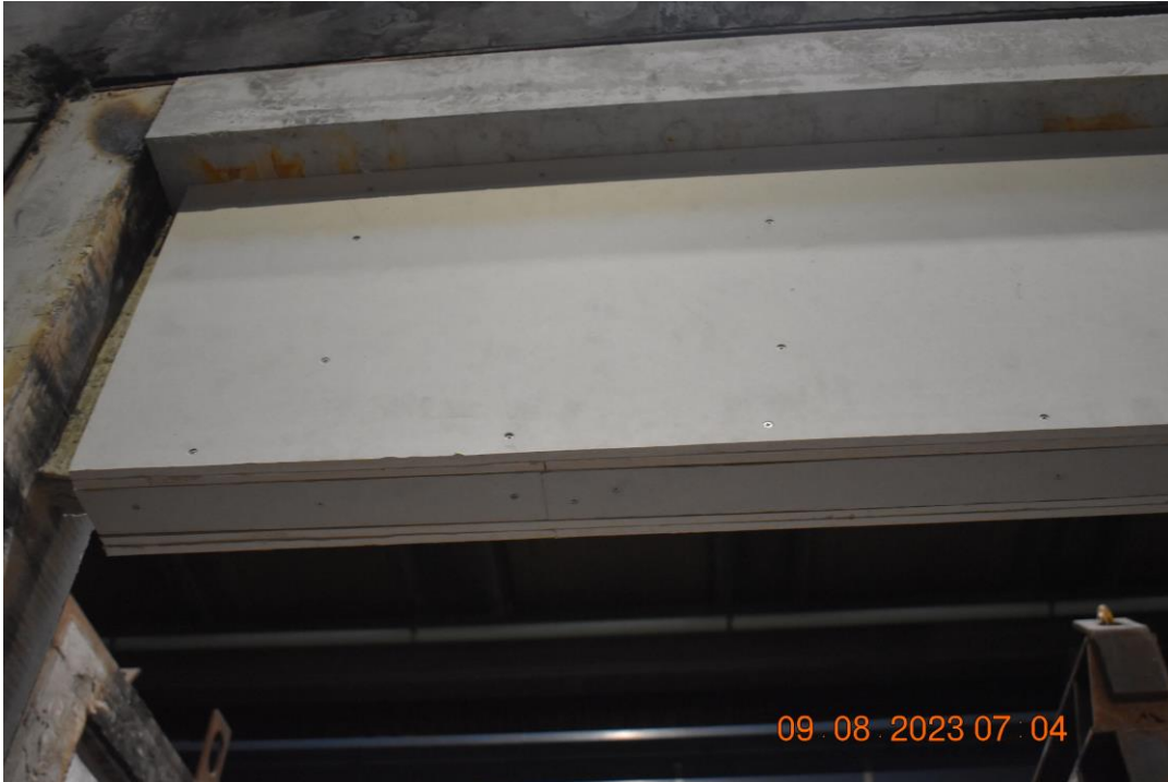
Photo No. 3 Fixed steel framework mounted with gypsum boards.
