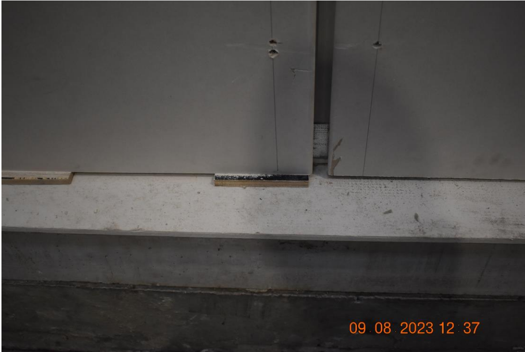
Photo No. 9 Prefabricated tongue and groove system, seen from outside the wall. connected to the testing frame.
