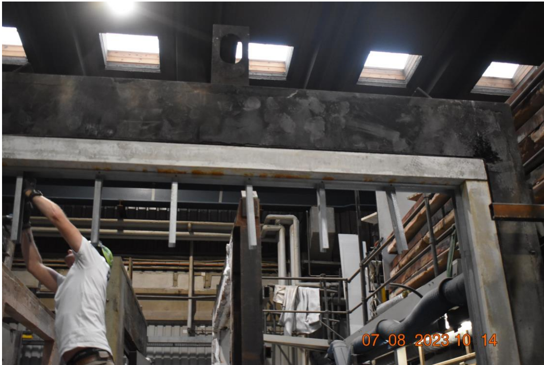
Photo No. 1 Mounting of fixed steel framework, top of specimen.
