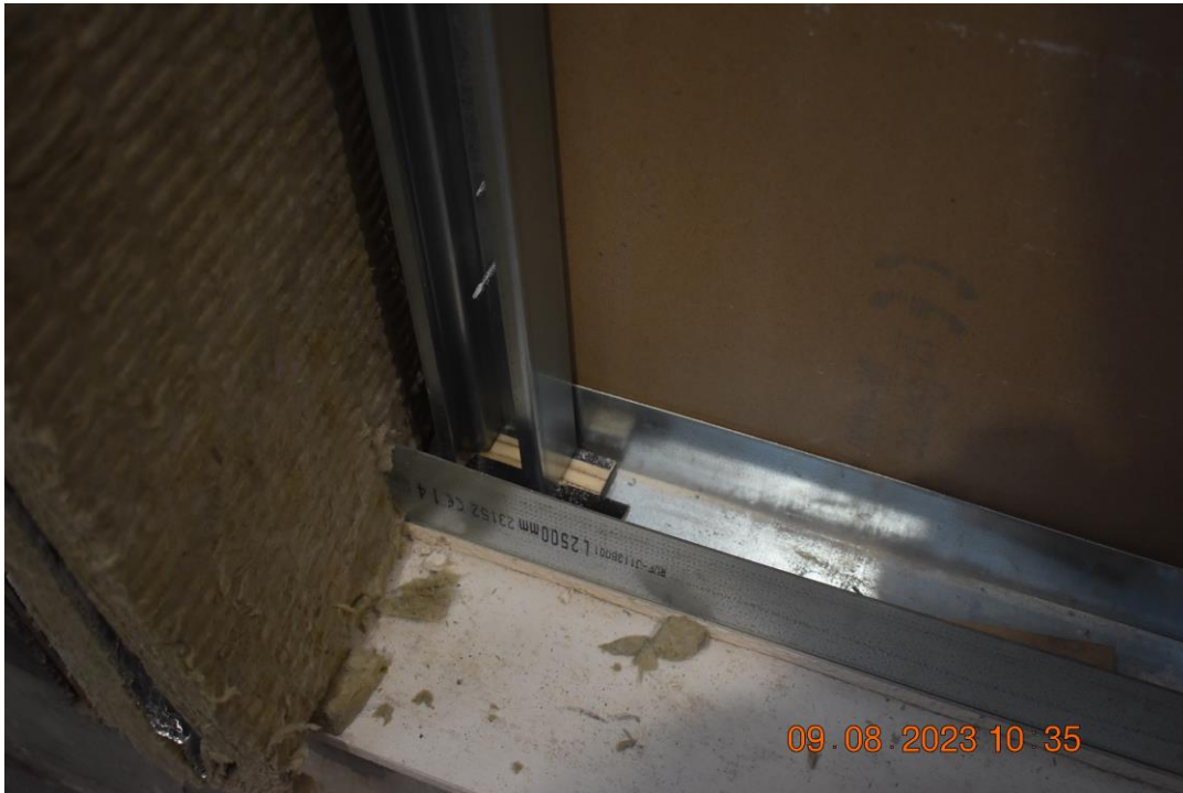
Photo No. 5 Mounting of prefabricated wall against free edge.
