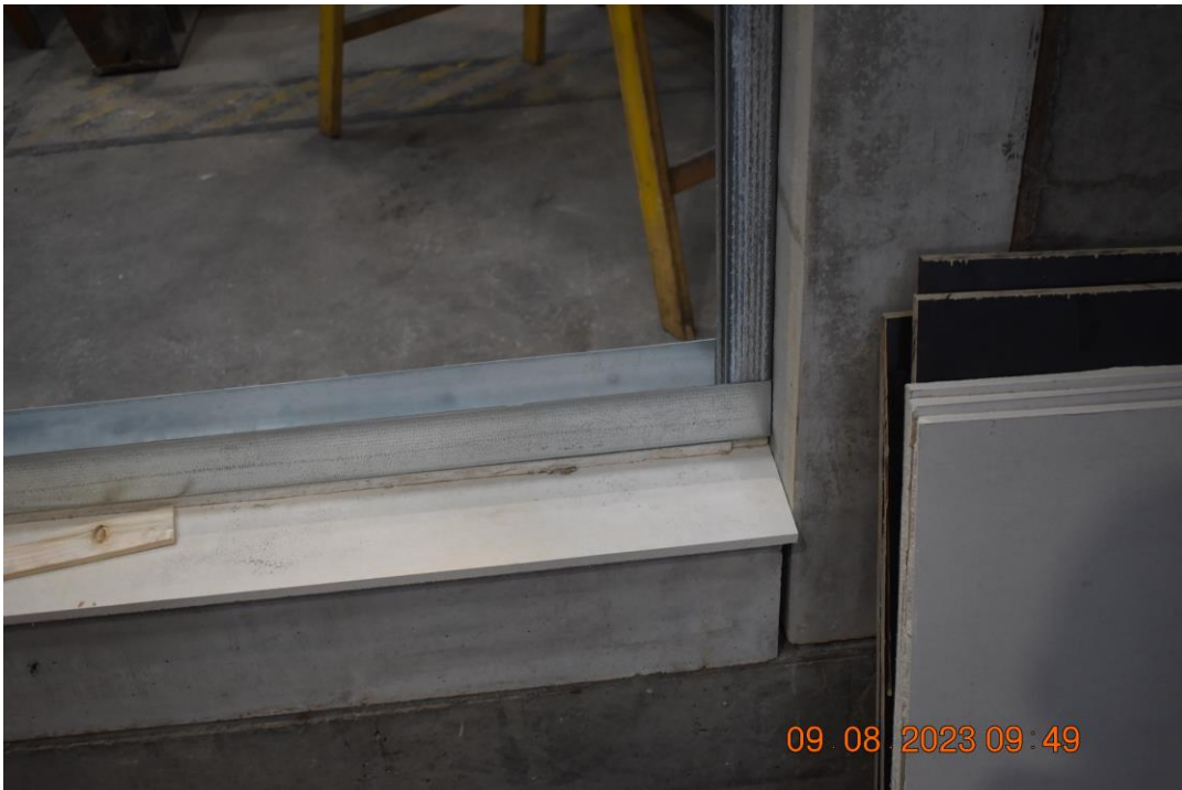
Photo No. 4 Bottom 70mm U-profile mounted to a calcium silicate boards and test frame.
