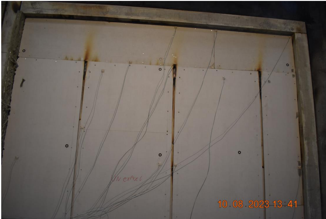
Photo No. 17 Test specimen after 64 minutes of testing.
